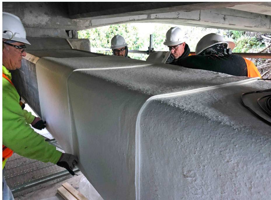
Cellulose fabric attached to concrete surface
