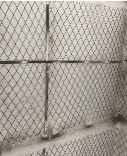
Titanium mesh with welded titanium distribution bar
