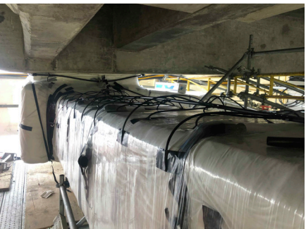
Cellulose matting wrapped in plastic sheet with drip hoses
